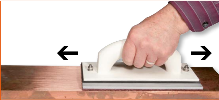
Cleaning process, busbar or surface cleaning
